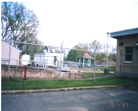
Village Waste Water Treatment Plant
