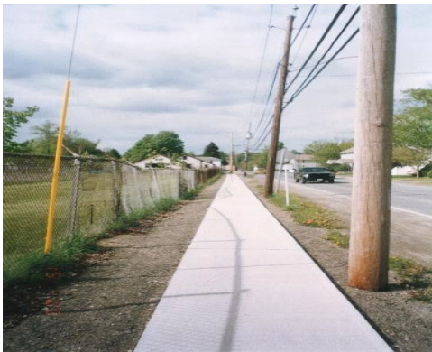
New Sidewalks on Church Street
